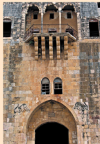
View of first floor balcony
